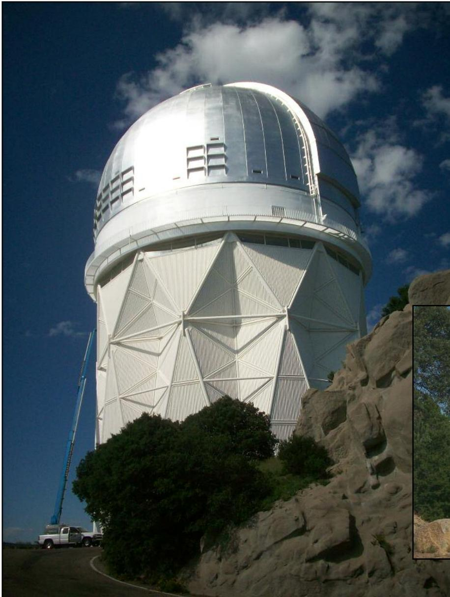
**A FLEXIBLE SILICONE COATING WAS APPLIED TO THE ROOF OF THE DOME. THE RADIANT BARRIER ROOF COATING SIGNIFICANTLY REDUCES EXTERIOR ROOF SURFACE TEMPERATURES.**
