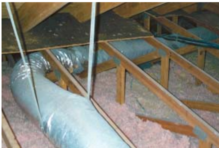
Figure 4. Radiant barrier foil under the rafters stops heat from radiating into the attic, because the foil will not emit heat radiation even when it's hot (top left and right, before and after). Lo/Mit low-emissivity silicone coating spray-applied to the roof underside (right) is a cost-effective alternative method.
