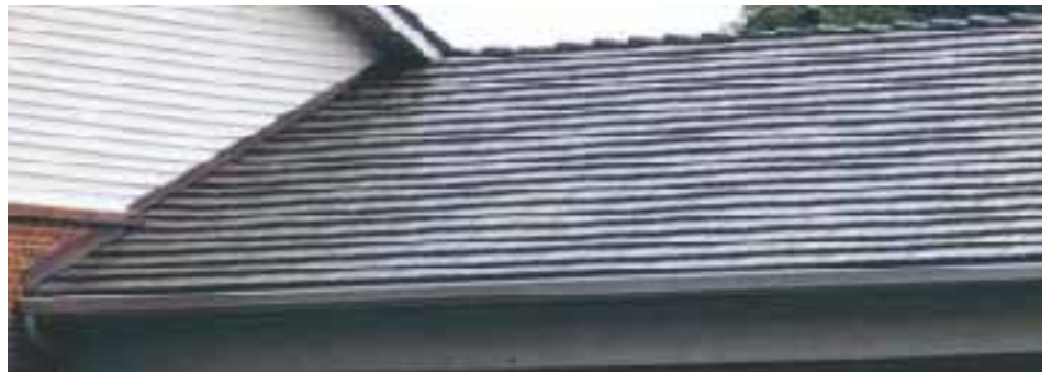
Figure 2. Kynar roof coatings using spectrally selective pigments from Ferro Corporation allow Classic Roofs to produce aluminum and steel shingles in several dark colors that meet Energy Star minimums with solar reflectances better than white asphalt shingles. Tests indicate that the colors will sharply reduce solar heat gain through the roof.
