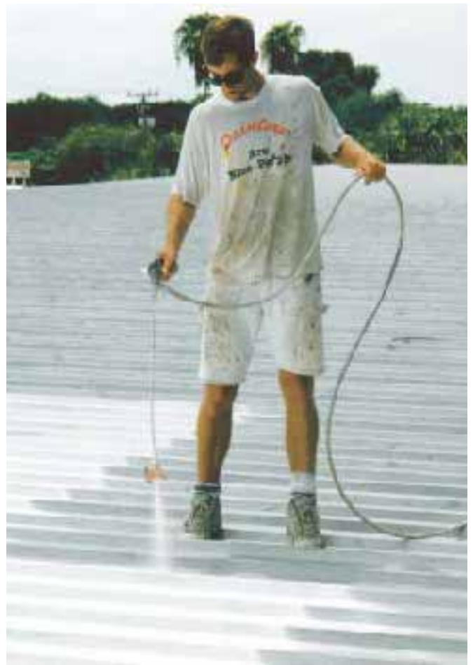
Figure 3. Unfinished galvanized steel roofs may look shiny when new, but they age quickly to become very nonreflective. The infrared thermal scan (above left) shows the drop ceiling (top) at a radiant temperature of almost 90°F under the metal roof of a strip mall building, despite insulation below the roofing. When FSEC researchers applied a reflective coating (right), the building’s air-conditioning power use dropped 16%, and tenants reported improved comfort. One tenant even called to thank the landlord for fixing the air conditioner. (He hadn’t.)
