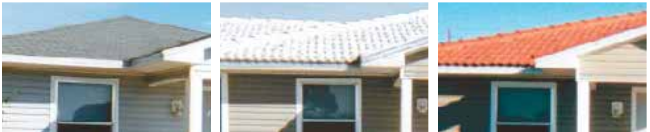
Figure 1. Florida Solar Energy Center researchers compared the air-conditioning power use of seven identically built houses with different roof coverings. Reflective roofing dramatically reduced total power use (bottom chart) and had an even greater effect on peak A/C power demand (middle chart). Insulating the roof deck and sealing the attic, without using a reflective roof, cut total energy use somewhat but did not reduce peak cooling loads noticeably.
